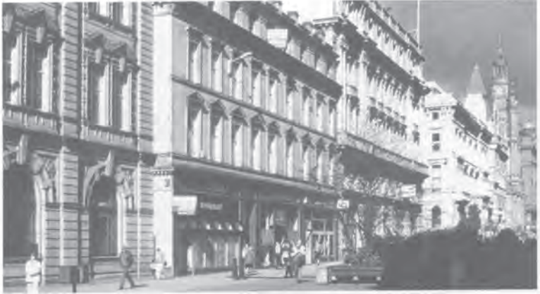
Buchanan Street, west side. From left to right (using the original building names): Royal Bank of Scotland (extension, A. Sydney Mitchell, 1886-8); not known; Carron Building, on the corner of St Vincent Street (James Boucher, 1884); Western Club (D & J Hamilton, 1839-42); Stock Exchange (John Burnet, 1875-7); the tower of St. George's Tron church (William Stark, 1807-9); Liberal Club (J. J. Burnet, 1886) and the Athenaeum Theatre (J.J. Burnet and J.A. Campbell, 1891-93).
