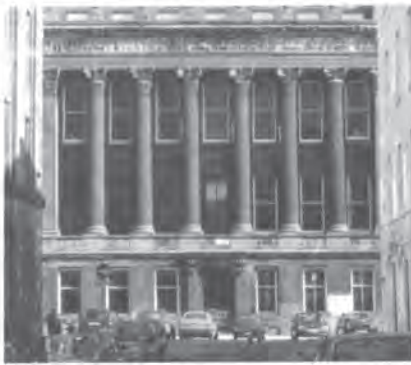
Top: Wilson Street with the pedimented portico of the City and County Buildings (Clarke & Bell, 1842-4). Bottom: Merchants' House (Clarke & Bell, 1842-4).
